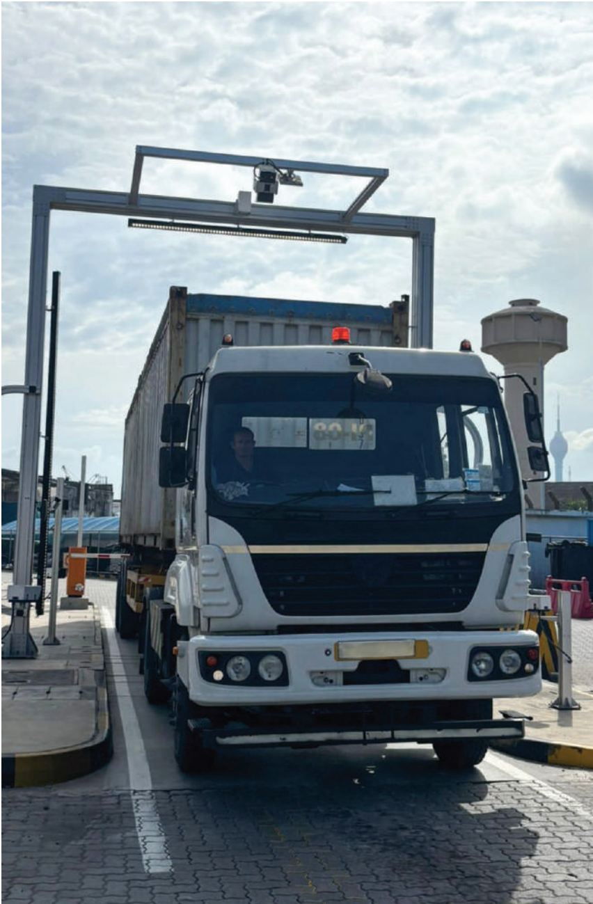
Steady progress in gate automation infrastructure, powered by Optical Character Recognition (OCR) technology.
