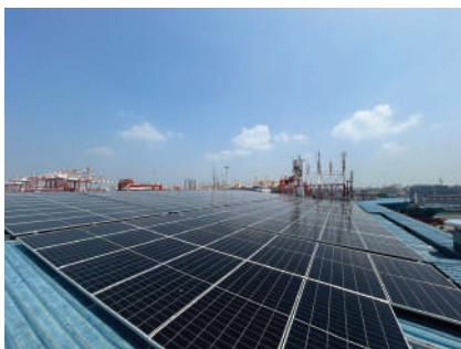
Installation of Rooftop Solar Panels
